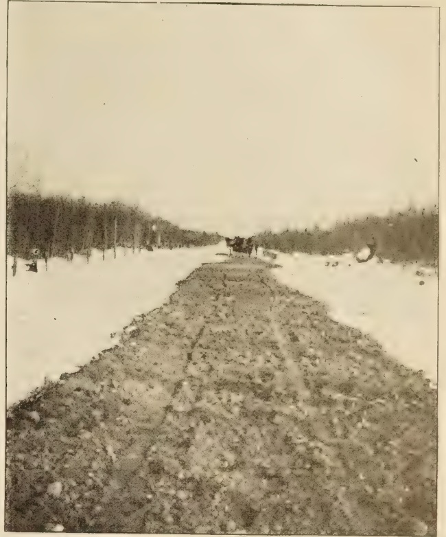
GRAVEL SURFACING PLACED IN WINTER, OCONTO COUNTY, WIS.
